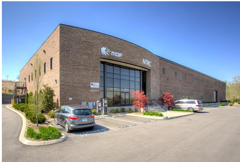
The HVA RoHAWKtics used to work at the MDF and NTRC buildings during build season. The team worked here six out of seven years.
